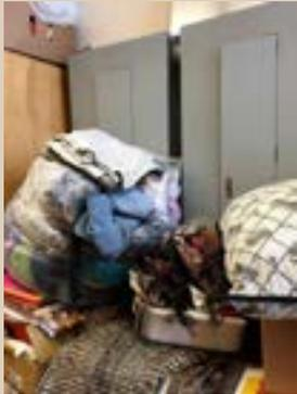
*Fire Code of NYS § 605.3 - A working space of not less than 30 inches in width, 36 inches in depth and 78 inches in height shall be provided in front of electrical service equipment. Where the electrical service equipment is wider than 30 inches, the working space shall not be less than the width of the equipment. No storage of any materials shall be located within the designated working space.*
